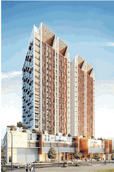
The development comprises two towers above a retail podium at Gosford.
